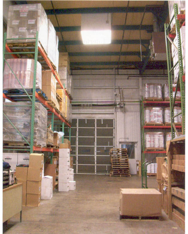
The skylights' appearance at night (right) is nearly identical to their appearance during the day (left) thanks to the fluorescent tubes behind the bottom diffuser.
