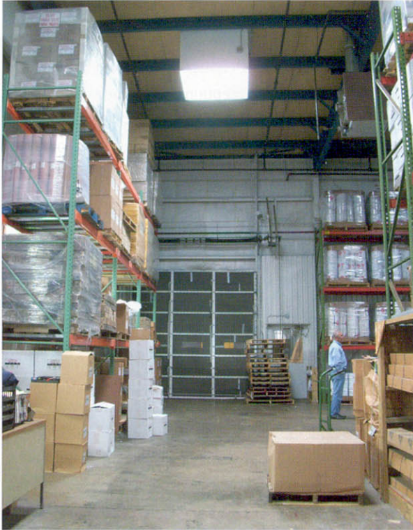
The skylights' appearance at night (right) is nearly identical to their appearance during the day (left) thanks to the fluorescent tubes behind the bottom diffuser.
